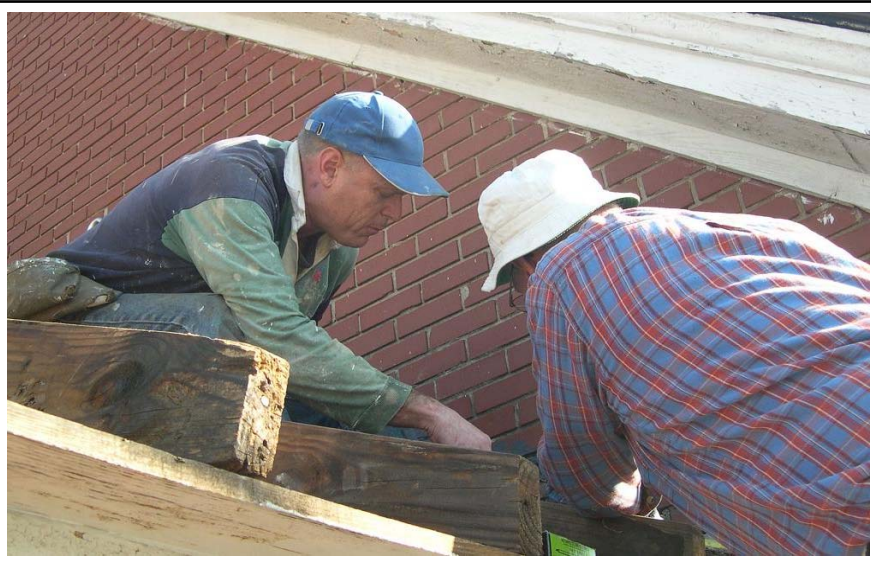
Bruce Herr and Doug Hattersley did roof repair.
